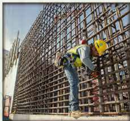
Rebar installation at the Highly Enriched Uranium Materials Facility
