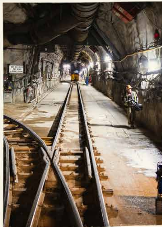
P Tunnel is used for seismic, acoustic, electromagnetic, and radionuclide experiments that inform nonproliferation and arms control initiatives
